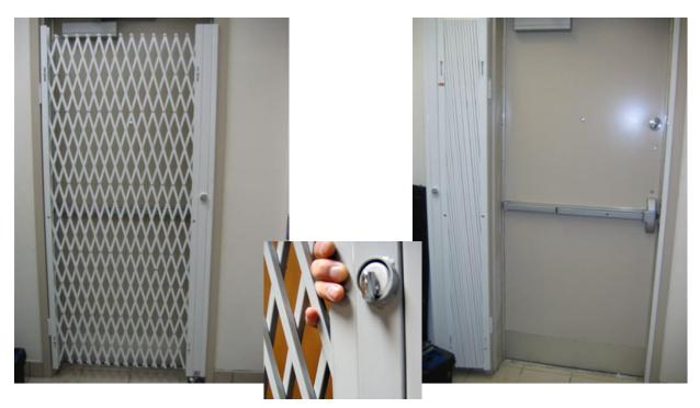
Double diamond webbing and the L206 locking post prevent the hands from accessing the thumb-turn when the security gate is in the locked position.
